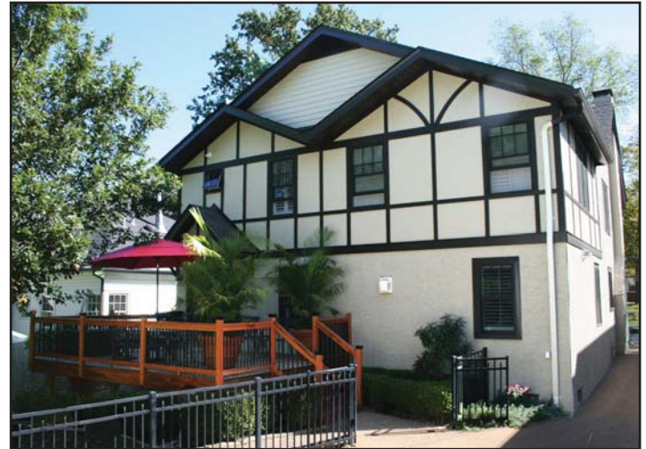
Rear After Addition
