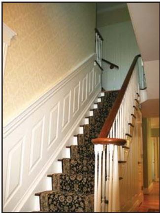
Wainscoating added to left wall of stairwell.
