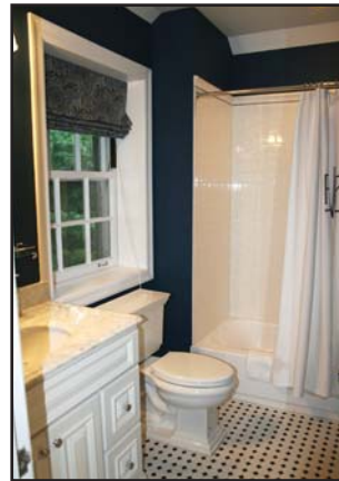
New tile, paint, and vanity replacement.
