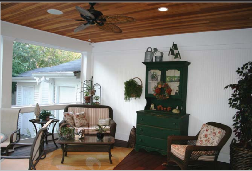
Maintenance-free screen porch features tongue and groove ceiling, bead-board walls, ipe wood floor and wide railings for plants and party drinks
