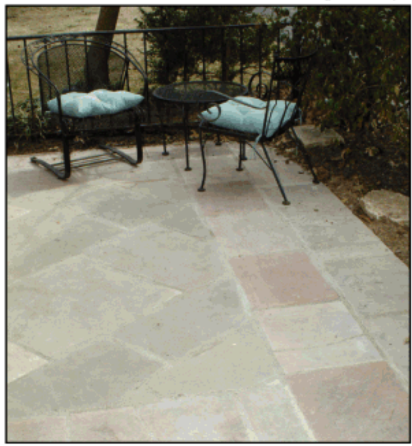
Existing stone from a dangerously uneven two-level patio was recycled to create a usable space alongside the house.
